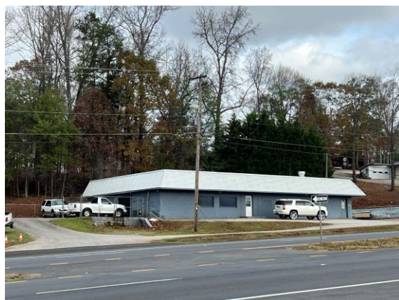
Parcels 13 and 14 are located at 3640 and 3642 Calhoun Memorial Highway within the Project Area.
