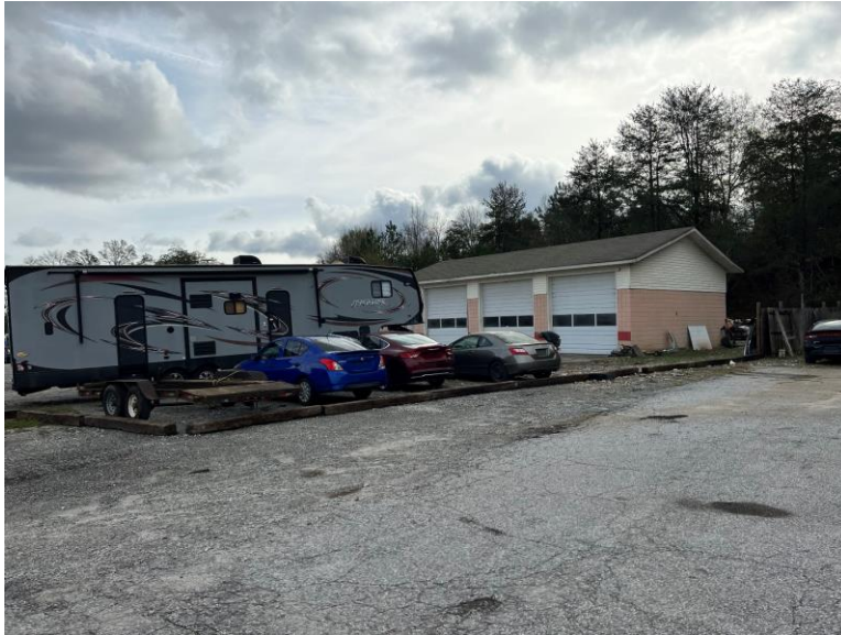
View of Parcel 21, City Auto Sales, 3725 and 3729 Calhoun Memorial Highway within the Project Area.
